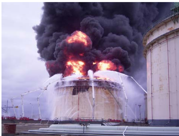
Figure 6. Tank fire occurred two days after the event (photo by Fire and Disaster Management Agency).
