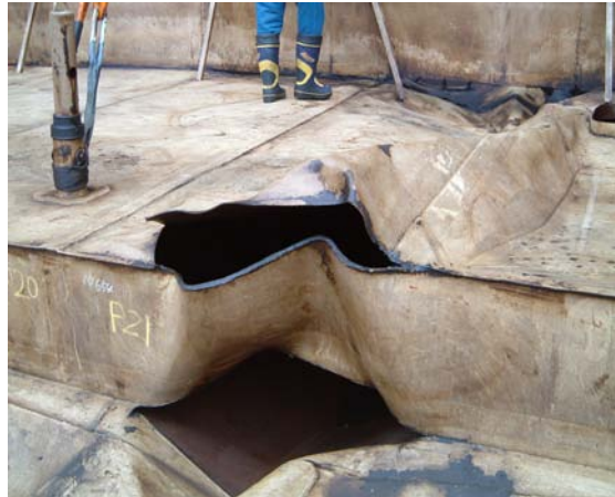
Figure 9. Failure of pontoon.
