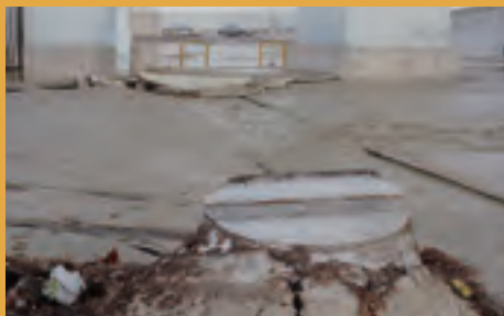
Manhole pushed up by liquefaction (Hyogo-Ken-nanbu Earthquake, 1995) (Photo provided by Takashi Tanikawa, Saitama University)
