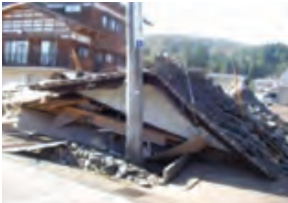
Collapsed wooden house (The Mid Niigata prefecture Earthquake in 2004) (Photo provided by Niigata Pref.)
