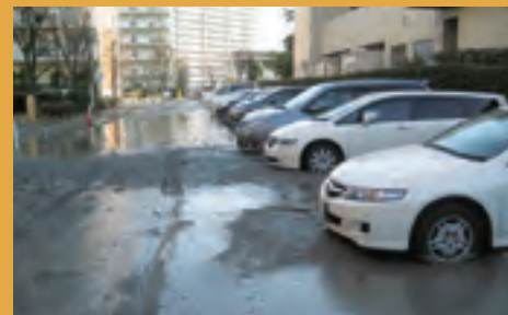
Gushed sand (The 2011 off the Pacific Coast of Tohoku Earthquake) (Photo provided by Tomioka Estate Home Management Association, Urayasu City, Chiba Pref.)
