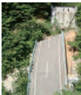
Collapsed Maturube Ohashi Bridge due to large-scale slope failure caused by the Iwate-Miyagi Nairiku Earthquake (Photo provided by South Wide-area Development Bureaus, Iwate Pref.)
