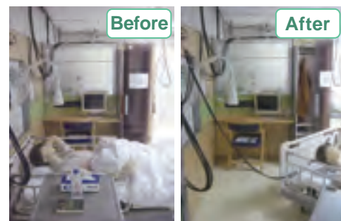
Inside the hospital with seismic isolation (Castor free beds moved significantly)
