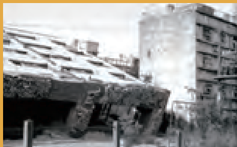
Building collapse due to liquefaction (Niigata Earthquake, 1964) (Photo provided by Toda Corporation)
